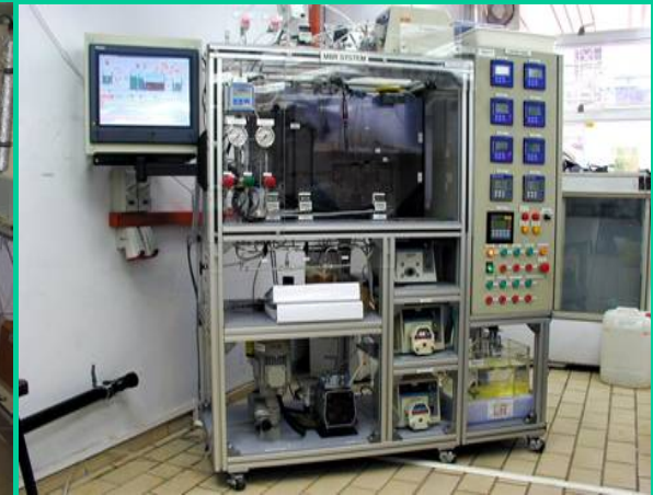
Membrane Bioreactor Water Reclamation System
